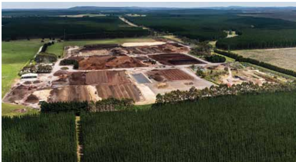
An aerial view of the Wandilo site.
