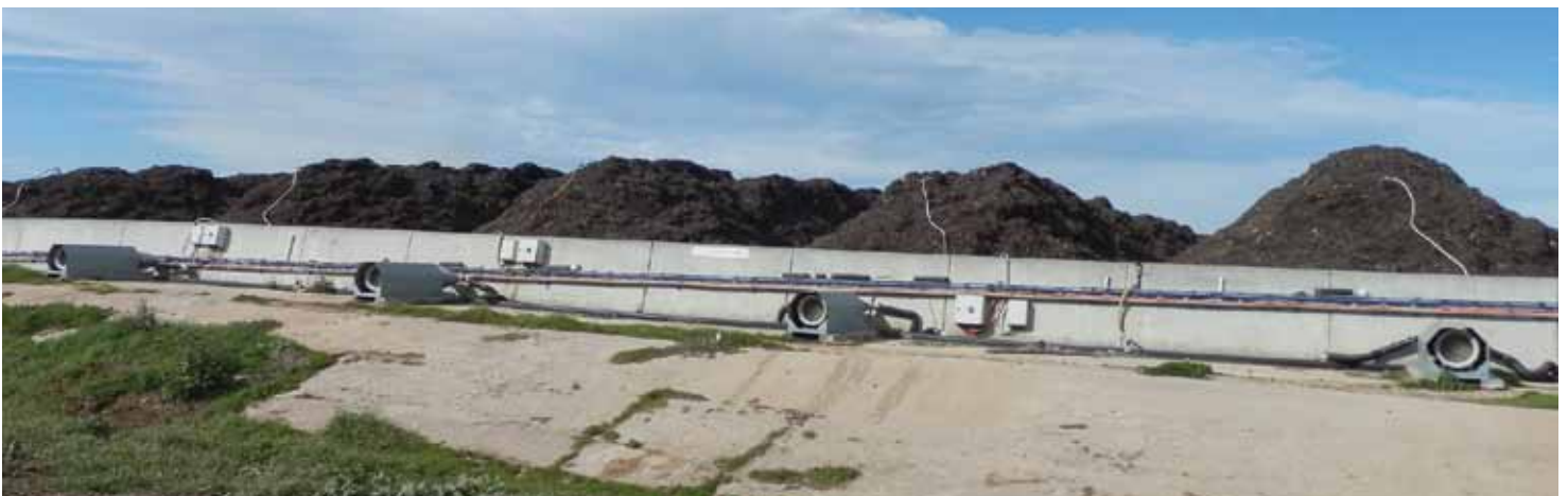
The forced aeration system does away with the need to turn the rows during the composting process.
